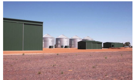
Shed & Silo Storage Setup
