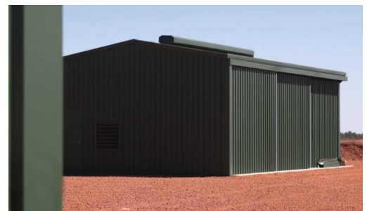
Vented Plant Shed (11m x 6m x 4m)
