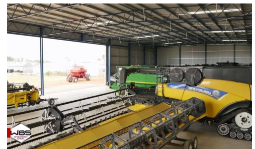
16mtr Clearspan Door Openings
